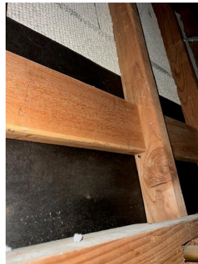
Plumbing chase interior
