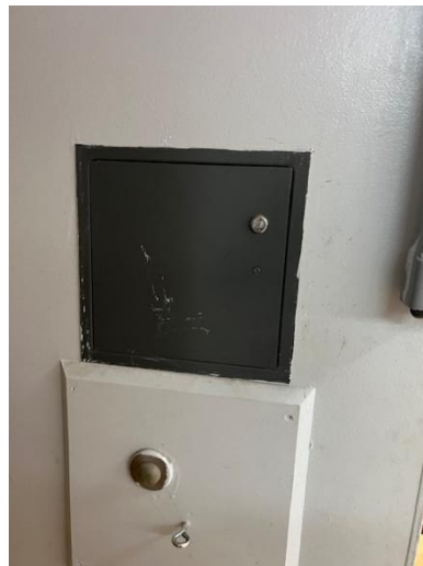
Plumbing Chase Access
