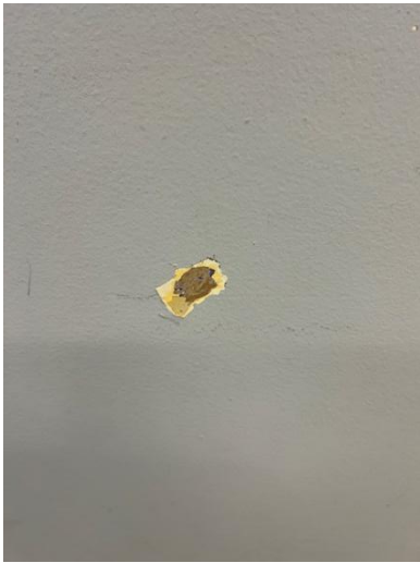
Rest room Paint
