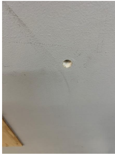
rest room wall
