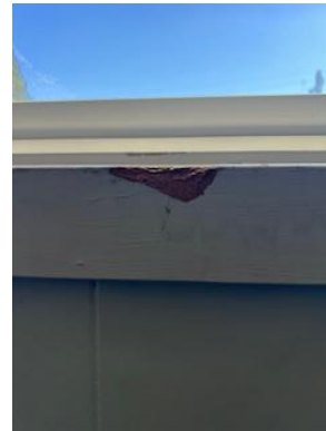
upstairs window sill
